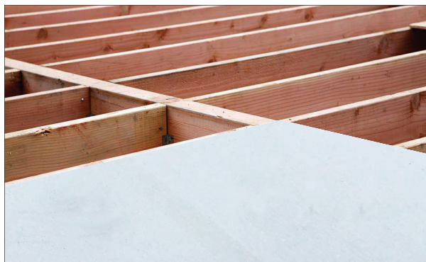
Subfloor over wood joists
