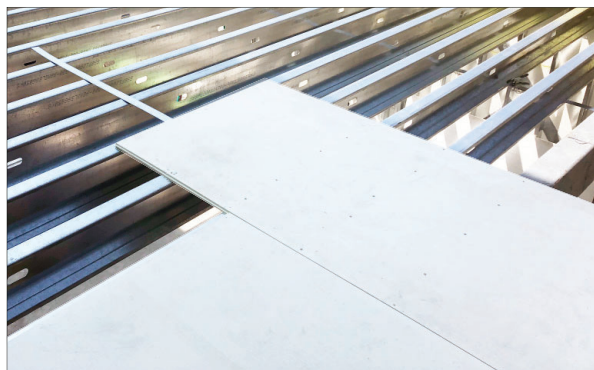
Subfloor over steel joists
